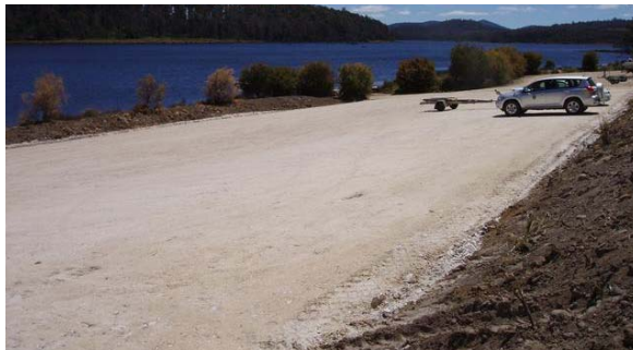
The new Improved car park at Four Springs Lake
