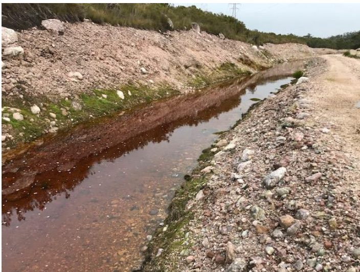
Tyndall Creek canal, the source of Tyndall Creek.
