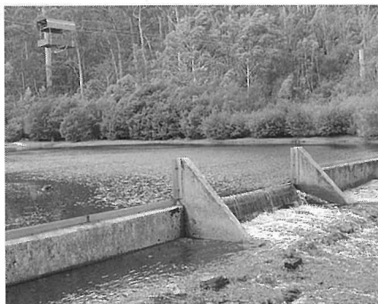
Ansons River Weir, north-east Tasmania
