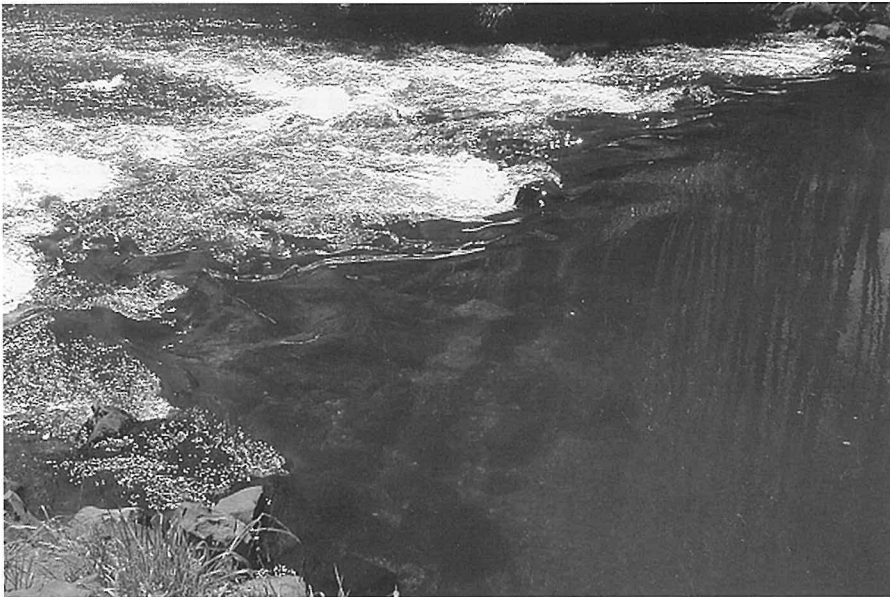
Cam River weir – the smooth flow over the submerged boulders (right half of picture) would make upstream passage of small fish difficult. Breaking up the flow with an array of large boulders that break the surface would make this barrier far more 'fish-friendly'.
