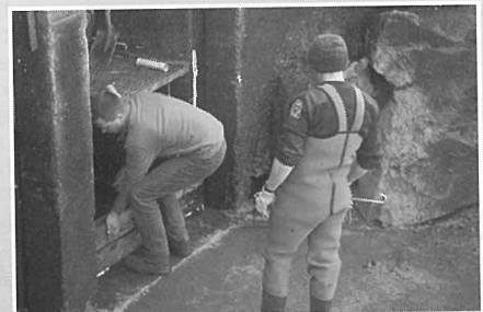
Sealing stop logs at the outflow gates from Lake Crescent. Photo Brett Mawbey
